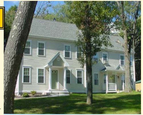
Woodridge Estate, new affordable homeownership in Woonsocket, RI sponsored NeighborWorks Blackstone River Valley. Project funded with NOP funds.
