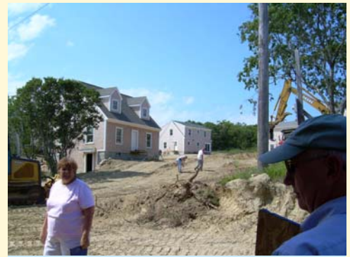
20 new affordable homes under construction in Block Island sponsored by Block Island Economic Housing Foundation. Project funded with NOP fund.
