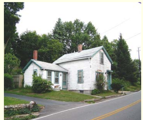
Pictures of a historic house in Westerly, RI that received lead hazard reduction treatment.
